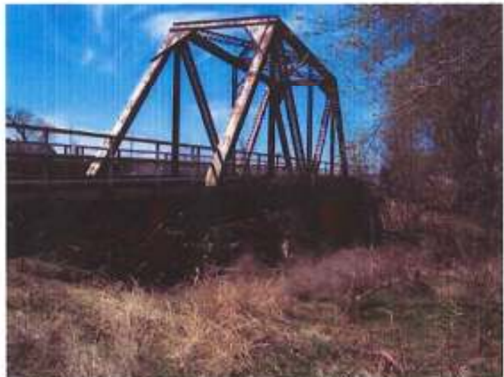
Figure 12: View of Union Pacific Railroad Bridge. Source: Brad Hus.
