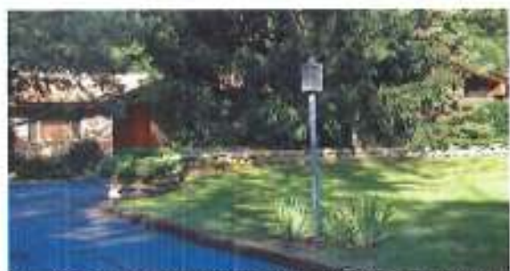
Fig. 25: Low flood wall for private residence. Source: NAI, 2003
